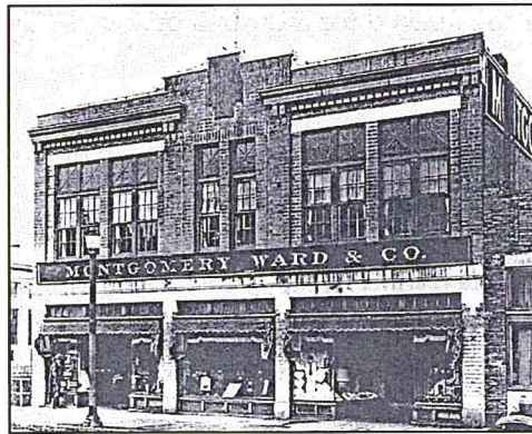
Figure 8: Commercial Building, Flat Roof Behind Parapet Wall
